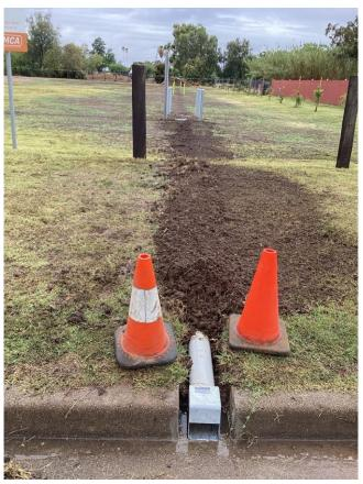
Figure 5 Drainage works showing the final connection to Chandos St kerb and pits in the background
