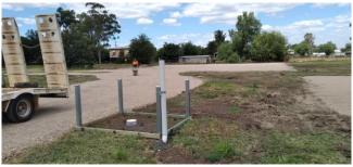
Figure 5 Form work for dump point at Gunnedah
