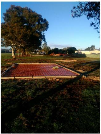
Figure 9 Form work for the shelter slab at Penola
