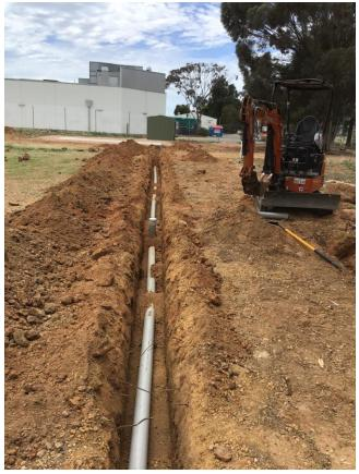
Figure 7 Trenching for plumbing works at Port Pirie
